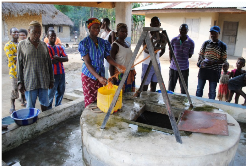
Wells built by RADA have transformed communities across Pujehun. Credit: Christian Aid
